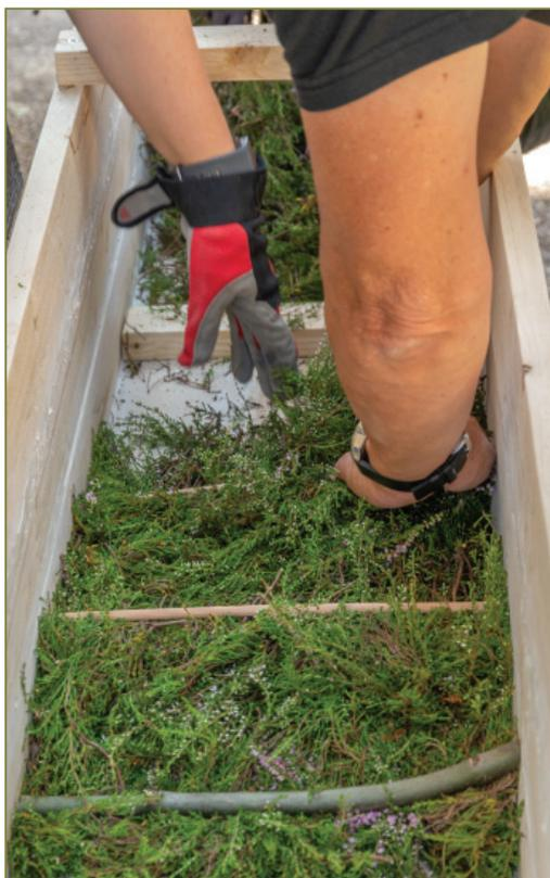
**Fig 7.** Lining the bottom of the sluice-box with heather and fixing it with thin wooden strips and twigs. Photo by F. Stremke
