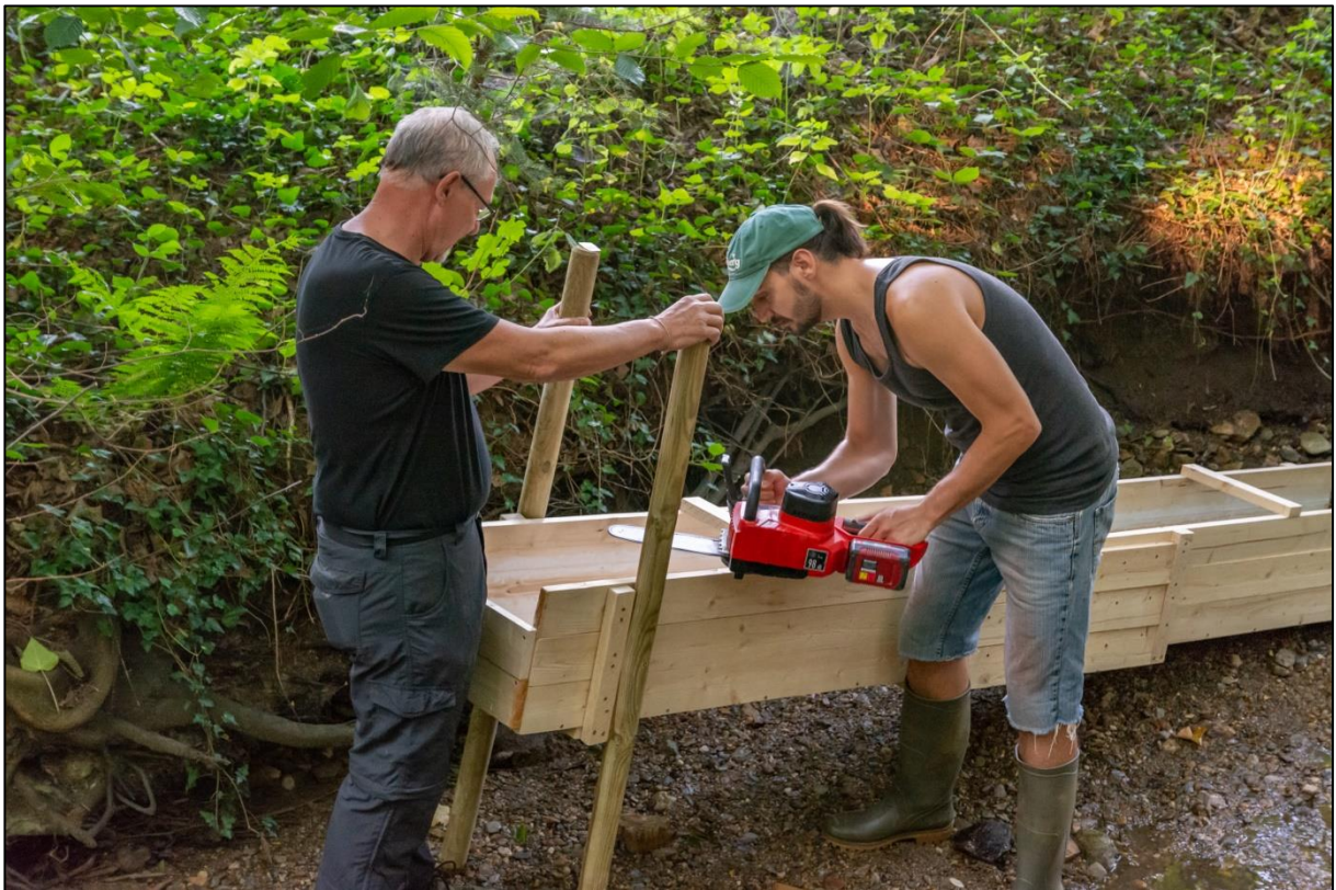
Fig 18. Mounting the sluice-box in the brook. Photo by F. Stremke
